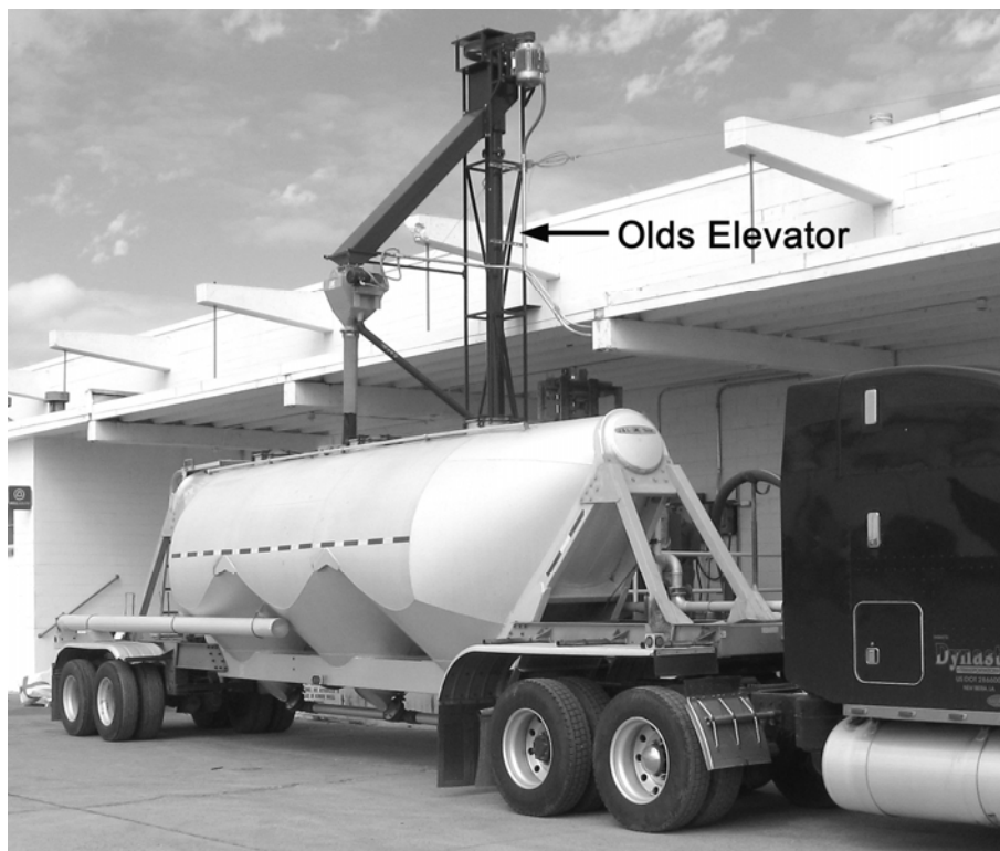
Figure 10 New Olds Elevator installed at Carbo Ceramics
